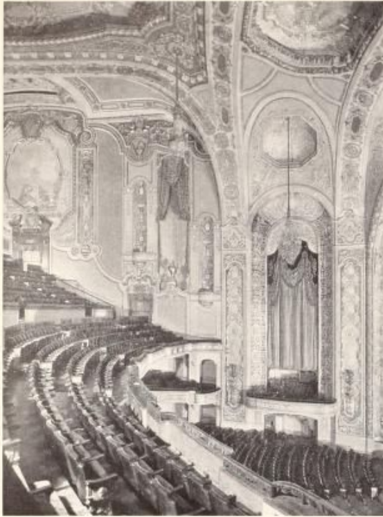
MICHIGAN THEATRE, DETROIT, SHOWING AUDITORIUM SIDE WALL AND ORGAN SCREEN TREATMENT C. W. & Geo. L. Rarr, Architects
