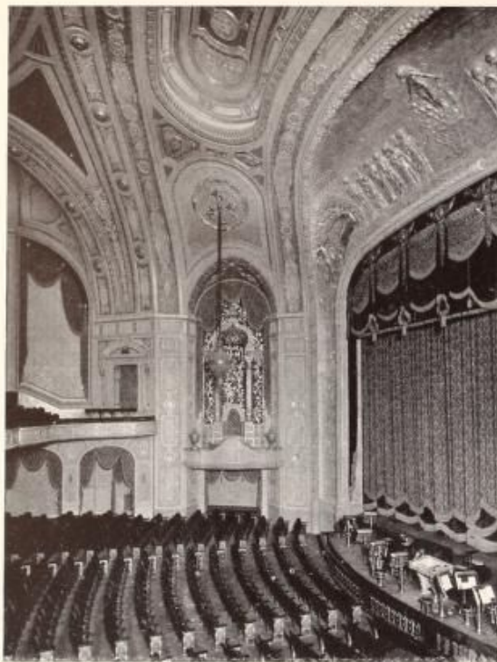
AUDITORIUM, SHOWING PROSCENIUM ARCH AND ORGAN SCREEN, RIALTO SQUARE THEATRE, JOLIET, ILL. C. W. & Geo. L. Rapp, Architects
